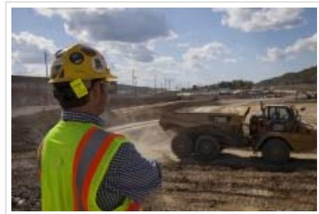
MyZone proximity detection system (as shown attached to the hard hat) alerts workers on the Uranium Facility Project when they are within 30 feet of heavy equipment.
